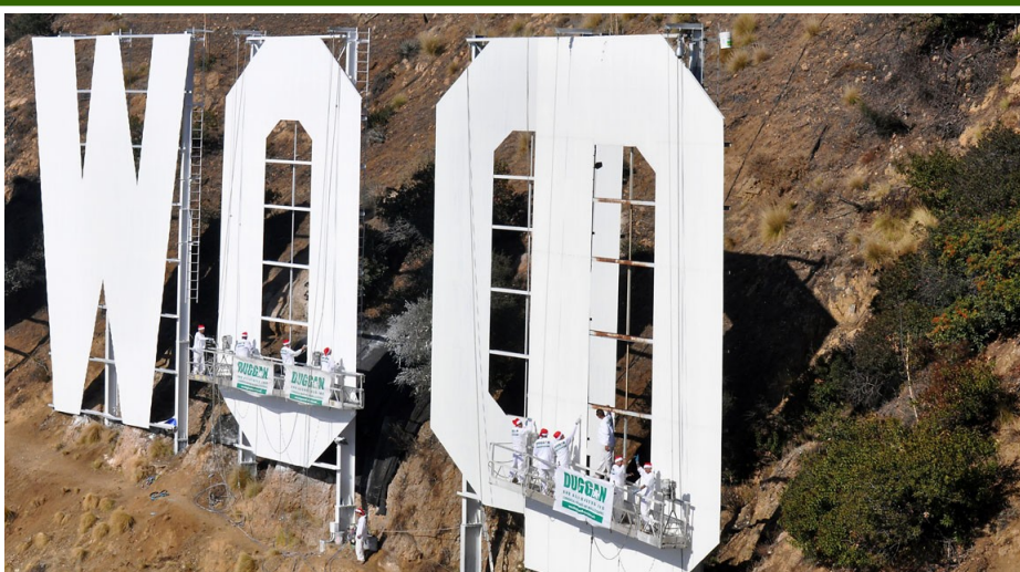
Hollywood sign is new again! Thanks to Duggan & Associates, H&E Equipment Services and Sherwin-Williams.
